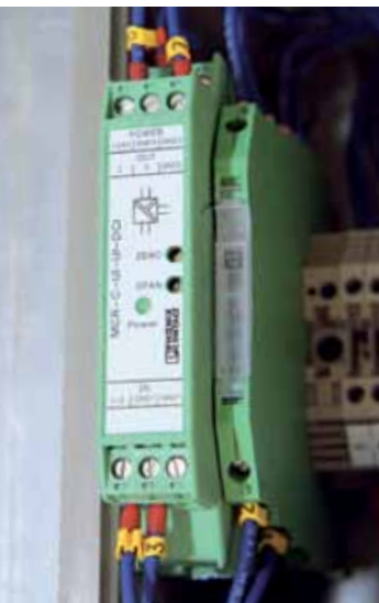
Signal transducer for conditioning the analog input signals.
